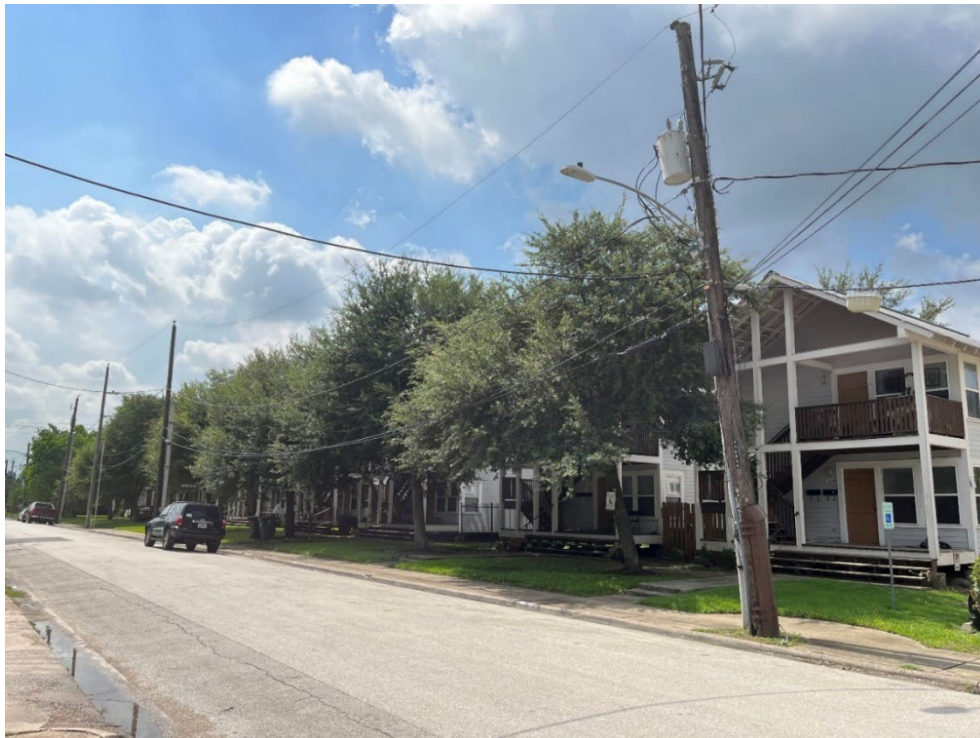
Figure 12 Duplex homes on Francis Street. Photo by the author.
