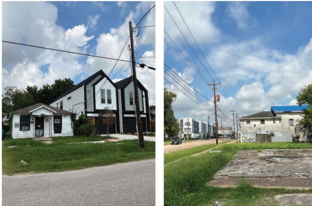
Figure 19 (left and right) New townhouse construction versus some existing residences and empty lots. Photos by the author.
