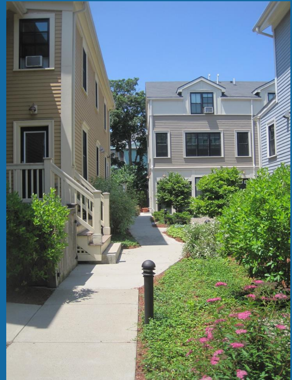
Columbia Court Apartments: 100% affordable development which involved a combination of new construction and historic preservation
