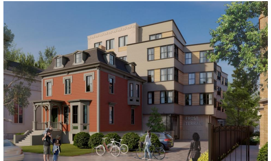
Frost Terrace: 40 affordable units approved by comprehensive permit, currently under construction
